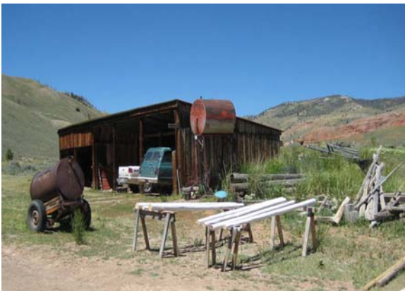
Working Ranch Assessment, WY
