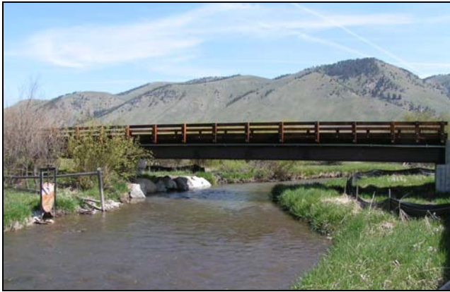
FLAT CREEK FISHING CLUB BRIDGE Teton County, Wyoming
