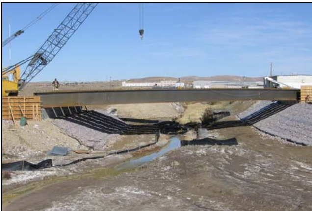
INDUSTRIAL DRIVE CONNECTOR KILLPECKER CREEK BRIDGE City of Rock Springs, Wyoming
