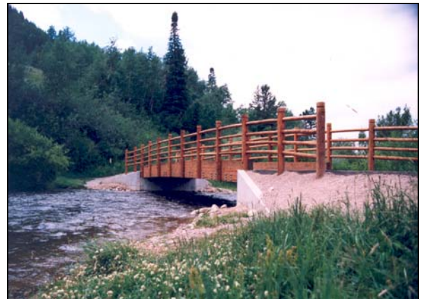
RUSS GARAMAN PATHWAY BRIDGE Teton County, Wyoming
