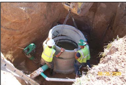
RURAL DEVELOPMENT/SLIB/LOCALLY- FUNDED SEWER MAINS REHABILITATION Dubois, Wyoming
