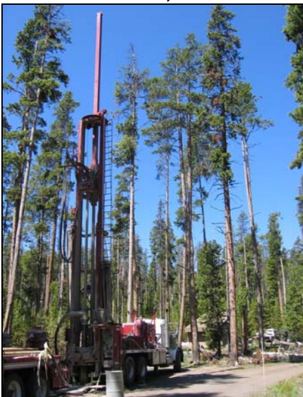
Fishing Bridge Water Supply Yellowstone National Park
