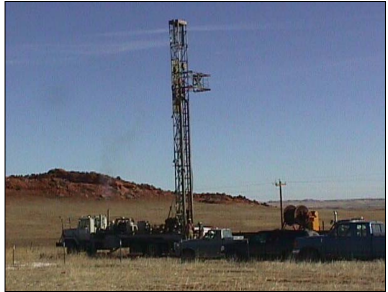
Well Testing & Pump Replacement Kaycee, WY
