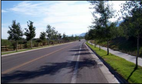
SNOW KING AVE. IMPROVEMENTS PROJECT Jackson, WY
