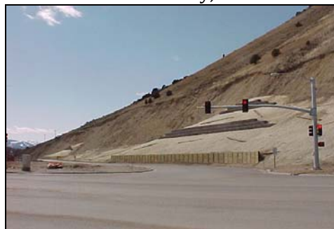
SOUTH PARK LOOP ROAD/HWY. 89 INTERSECTION Jackson, WY
