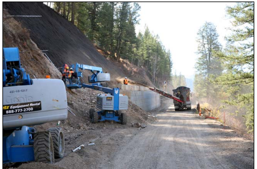
RETAINING WALL AND ROAD Teton County, WY
