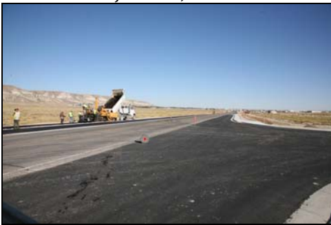
INDUSTRIAL DRIVE CONNECTOR Rock Springs, WY
