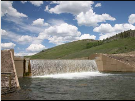
DAM ON LABARGE CREEK Lincoln County, WY
