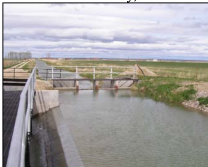
DIVERSION STRUCTURE, EDEN CANAL Sublette County, WY
