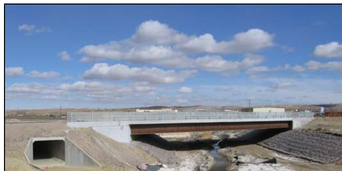
KILLPECKER CREEK BRIDGE Rock Springs, WY Hydraulic modeling, floodplain permitting, and scour analysis
