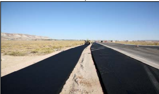
PATHWAY AND ROAD RESURFACING Rock Springs, WY
