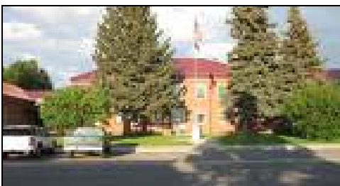
SUBLETTE COUNTY COURT HOUSE Pinedale, WY
