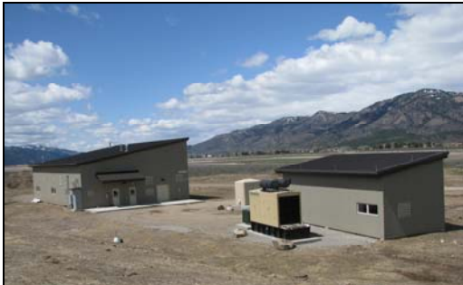
ALPINE WASTEWATER TREATMENT PLANT Alpine, WY
