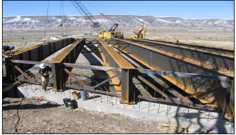
INDUSTRIAL DRIVE BRIDGE Rock Springs, WY
