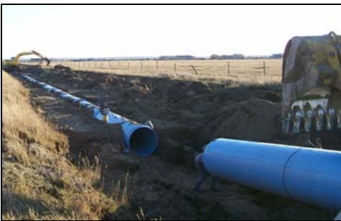
Ditch-to-Pipeline Conversion Project Eden Valley Irrigation District, WY
