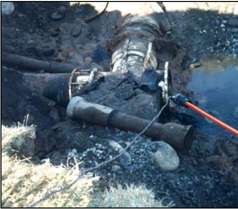
Lander Water Supply Project Lander, WY Jetting and cleaning 16" transmission line
