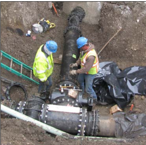
Teton Village Water & Sewer District Transmission Main Project Teton Village, WY
