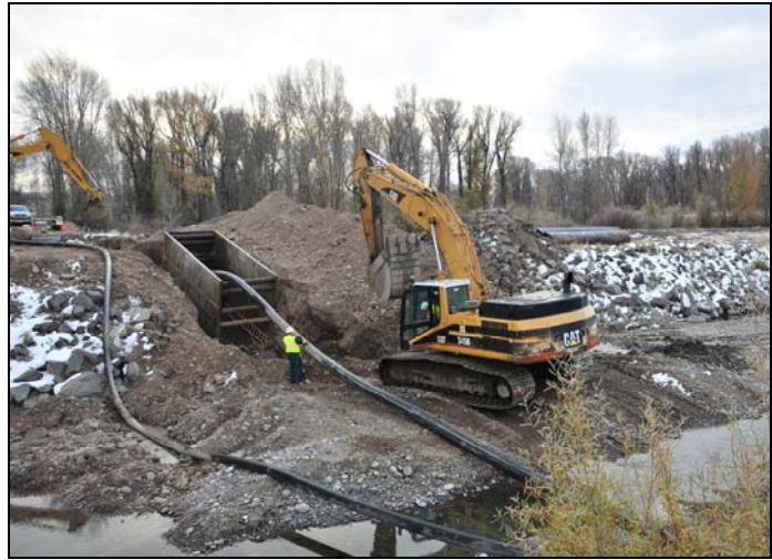
Wilson Sewer Project Teton County, WY
